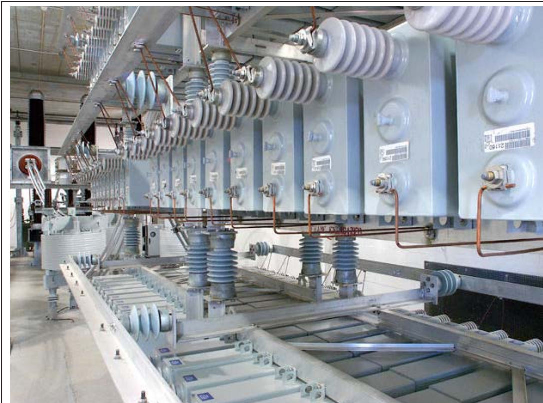
Photo: Siemens This static var (volt-ampere reactive) compensator on the Danish island of Lolland helps stabilize the low-power transmission system in the south of Denmark. Maintaining a stable grid has been a high priority with the widespread deployment of intermittent wind-generated electricity throughout the country.
